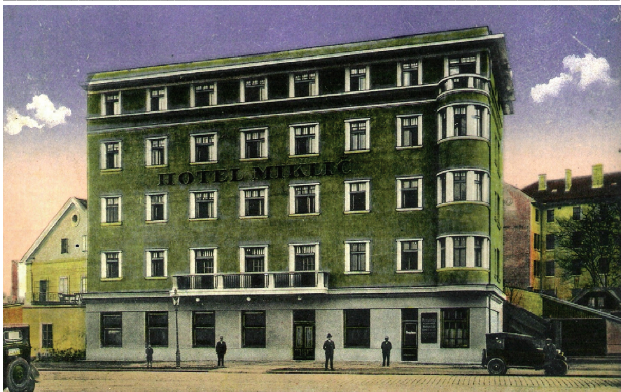
Slika 1. Hotel Miklič, gradnja I. faze (v ozadju levo hotel Južni kolodvor), leta 1928. Fig. 1. The Hotel Miklič, a construction of the 1st phase (in the background left is the hotel The south railway station) in the 1928th year.
