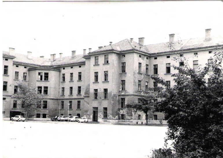
Fig.2,3. The Appearance of the »Domobranska« barracks from the yard, the 2nd phase, in the 1899th year
