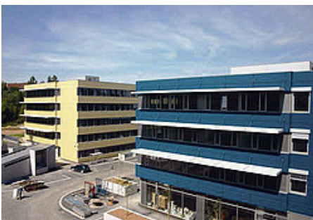
New business support centre buildings, Ljubljana
