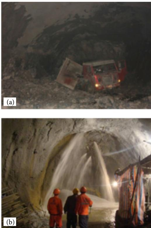
**Figure 1.** Rock-burst and water-gushing problems in deep buried hard rock in the Jinping II hydropower station: (a) strong rock burst (b) high-pressure and large-volume groundwater infiltration.[2].
