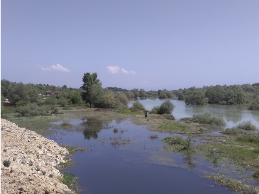
Figure 1. Location of water traps on Beli Drim, which had apparently been flooding.
