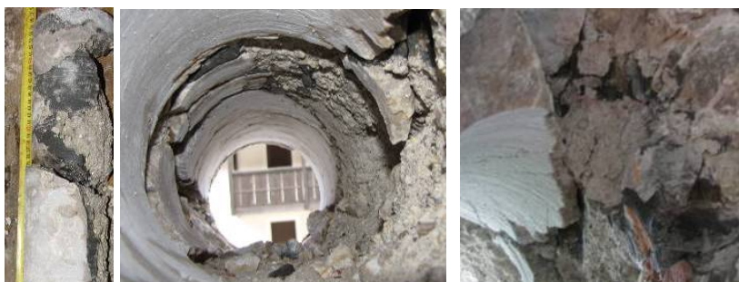
Slika 5.38: Jedro, vrtina in globinska sonda izvedena v zgornji polovici zidu 4-C2 Fig. 5.38: Core, borehole and in-depth probing at upper half of the wall 4-C2
