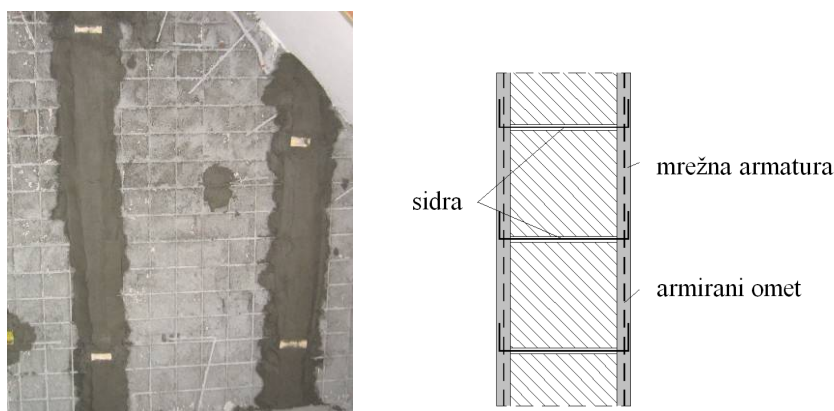
Slika 2.30: Primer utrditve opečnega zidu z armiranim ometom Fig. 2.30: Strengthening of a brick masonry wall with reinforced coating
