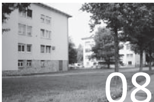
Stanovanjski bloki_ 1956–62_ Ulica Štefana Kovača 1-21
