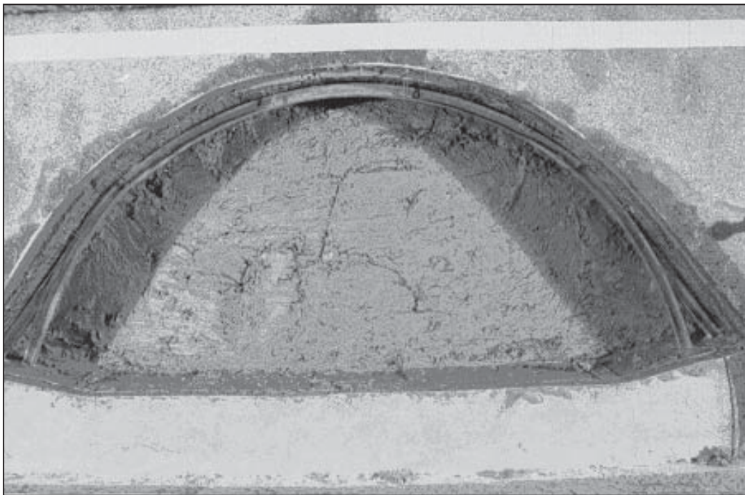
Figure 5. Installation of steel arches.
