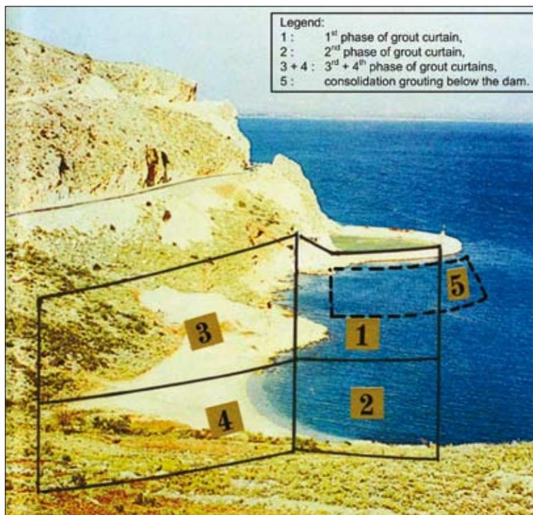
Fig. 16: Kiveri dam. Desalination structures proposed (2008, photo Breznik 1969).
