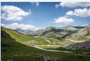
Bosnian mountain Visočica, Optical cable installed 10 years ago
