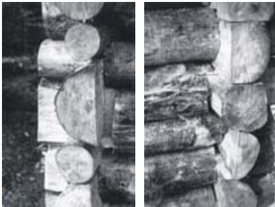
Slika 8, 9, 10: Primer novega senika in detajlov izvedbe na planini Trstje (foto: J. Kušar). Example of a new hayloft on the Trstje Mountain and construction details.
