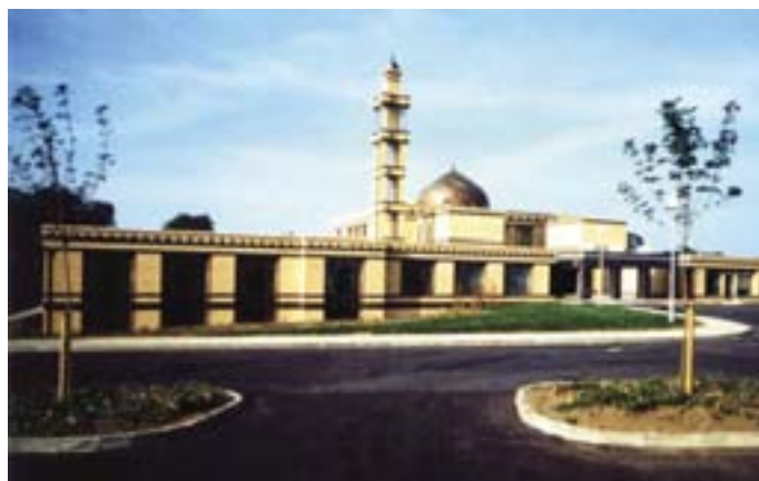
Slika 11: Mošeja v Dublinu, pogled celote [vir: Richardson, P., 2003: 157]. The mosque in Dublin, view of the complex.
