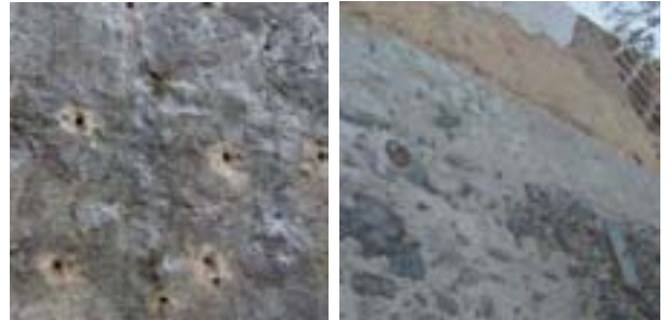
Slika 7: Zunanji zid: (a) injektiranje; (b) sidranje v ploščo. The outer wall: (a) injecting; (b) anchorage.
