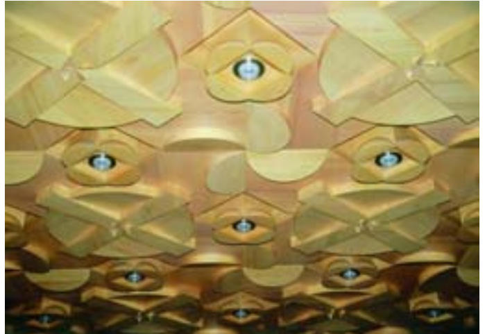
Slika 3: Izmenjajoče ponavljanje motivov in minimalni višinski zamiki ustvarjajo dinamično polnost ter plastičnost površine, le-ta pa povezuje bočna pasova poslikav v harmonično celoto. Strop je izdelan iz masivnega češnjevega lesa v naravni barvi. The consecutive repetition of motifs and minimal vertical shifts create a superficial dynamic fullness and plasticity, which link with the illuminated side panels into harmonic unity. The ceiling is made of massive cherry wood in natural colouring.
