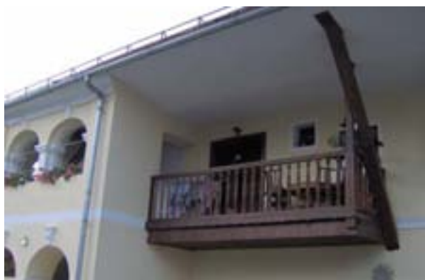
Slika 9: Objekt po delni prenovi: gank The building after partial renewal: "gank".
