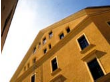
Slika 1: Masiven značaj fasad mlina je ohranjen. The massive character of the mill elevations has been preserved.
