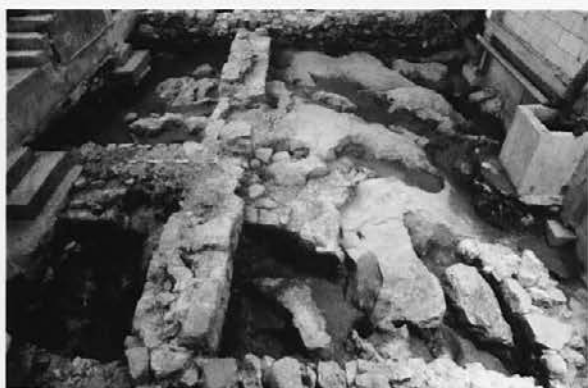
Fig. 8: Črnomelj - Pastoralni center: general view of the site after excavation - the Late Roman defensive wall and rectangular tower are in the foreground.
