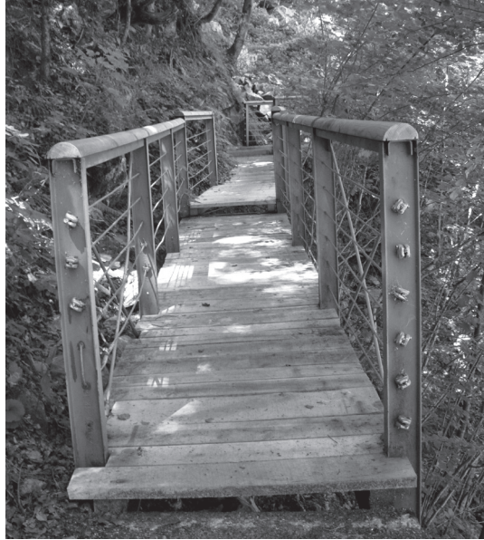
Slika 12: Konzolni mostički po obnovi leta 2013 Figure 12: Cantilever bridge after restoration in 2013
