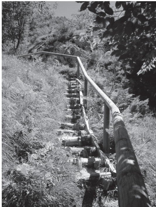
Sliki 18: Stopnice na strmi Bencetovi poti so varovane z leseno ograjo. Figure 18: The steps on the steep Bence Trail are protected by a wooden fence.
