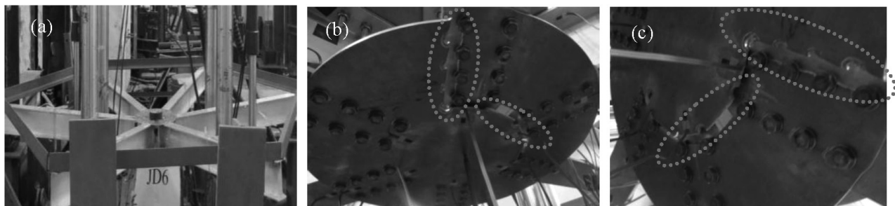
Figure 4: Traditional joint (JD6) failure mode: a) overall deformation, b) and c) shear failure of the lower cover plate
