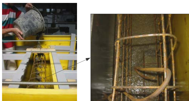
Slika 3.15: Večfazno vgrajevanje SCC mešanic v laboratoriju Fig. 3.15: Multi-layer casting of SCC mixtures in the laboratory
