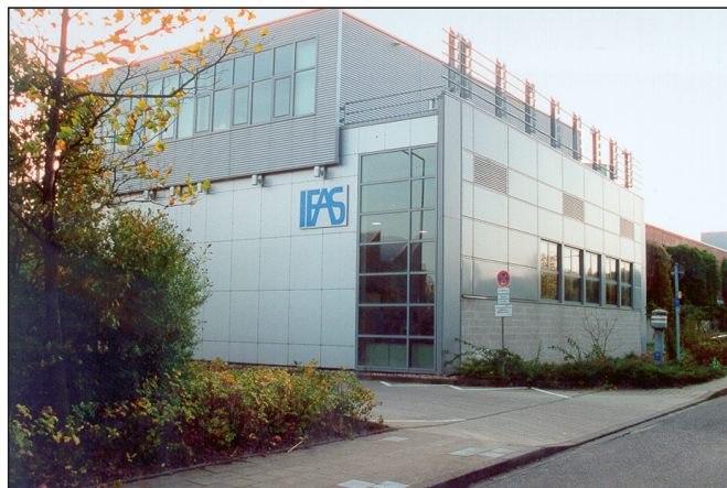
IFAS – Main building
