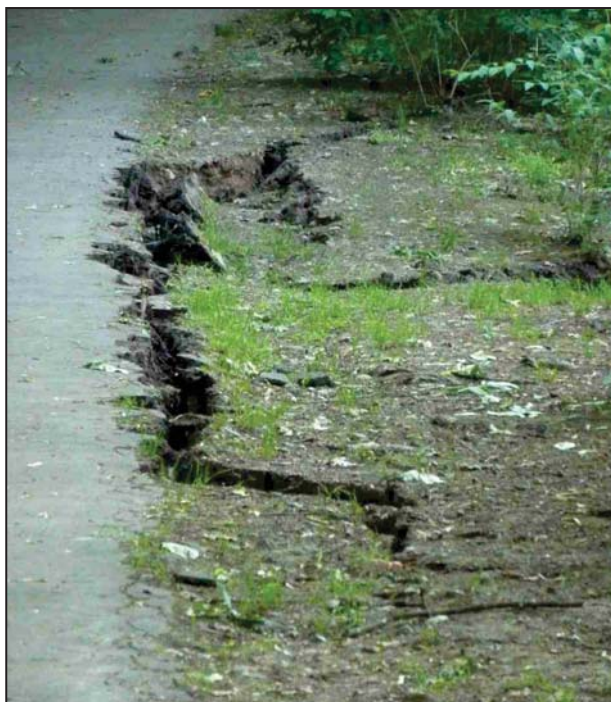
Figure 2. Tensile crack at the upper part of a slope.
