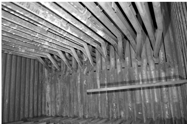
Figure 1: Part of superheater P1 and the membrane wall Slika 1: Del super grelca-pregrevalnika P1 in stena membrane
