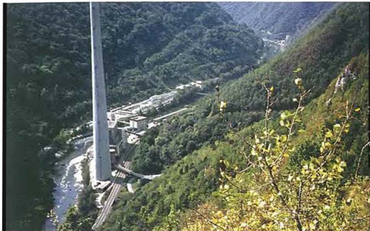
Slika 2: Termoelektrarna Trbovlje Figure 2: Trbovlje steam power station
