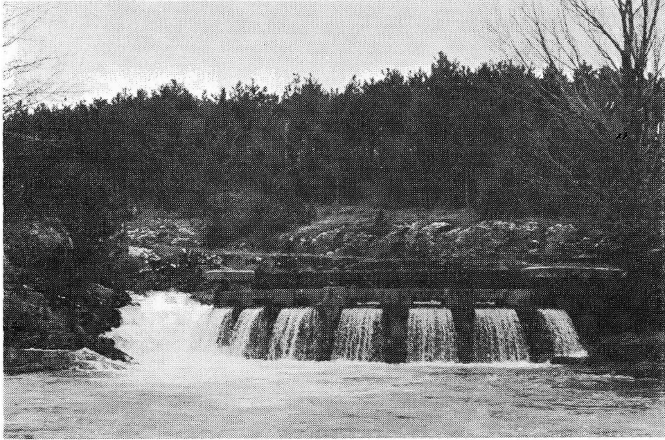
Sl. 4. Izvir Rižane, vodovodno zajetje zalito ob visoki vodi. Fig. 4. Rižana spring, water intake for public supply flooded after several heavy rains.
