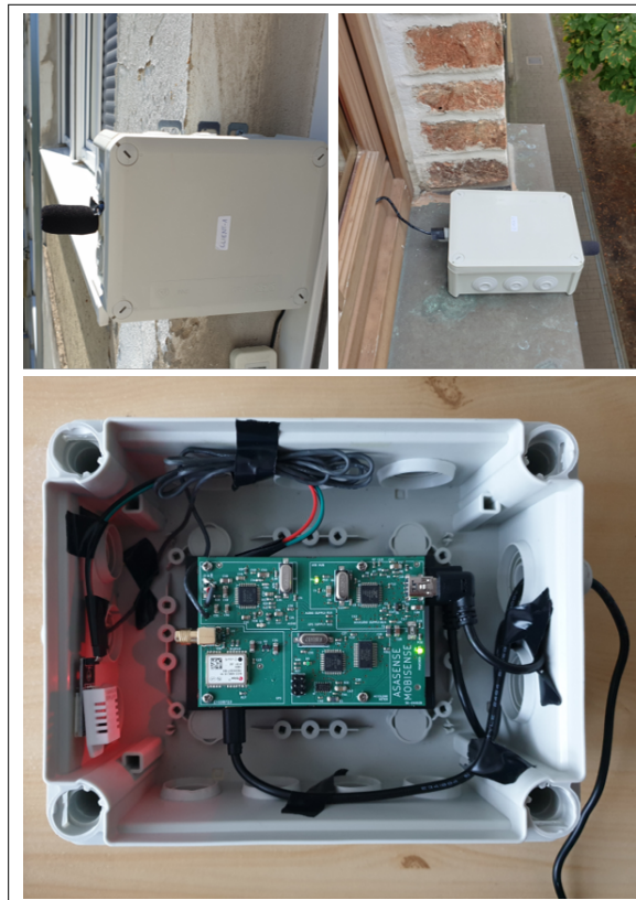
Fig. 2. Top: placement of sensor nodes on external building envelope. Bottom: operational setup of the sensors (microphone, temperature and humidity sensor, sound and vibration acquisition board) connected to a single-board computer (Raspberry Pi 3 Model B+).
