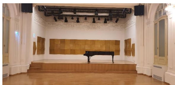
Fig. 14. The stage after installation of diffuser elements.
