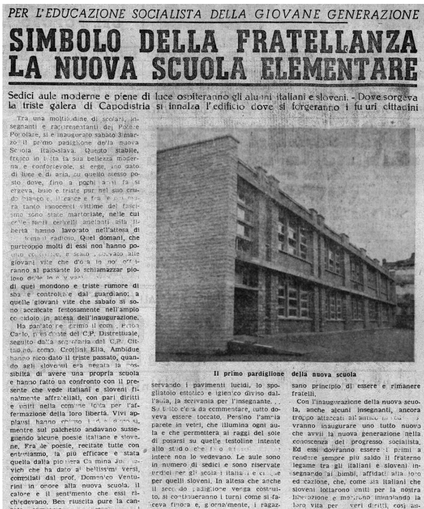
Figure 1: Ervinio Velušček, New Italian-Slovene elementary school (later elementary school of Janko Premrl Vojko) in Koper, 1948–1951 (source: La nostra lotta (a), 1951).
