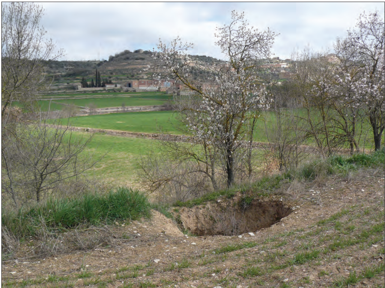
Figure 4: Piping connected to the soil surface behind a stone wall. In the background, valley floor terraces on El Sió floodplain.
