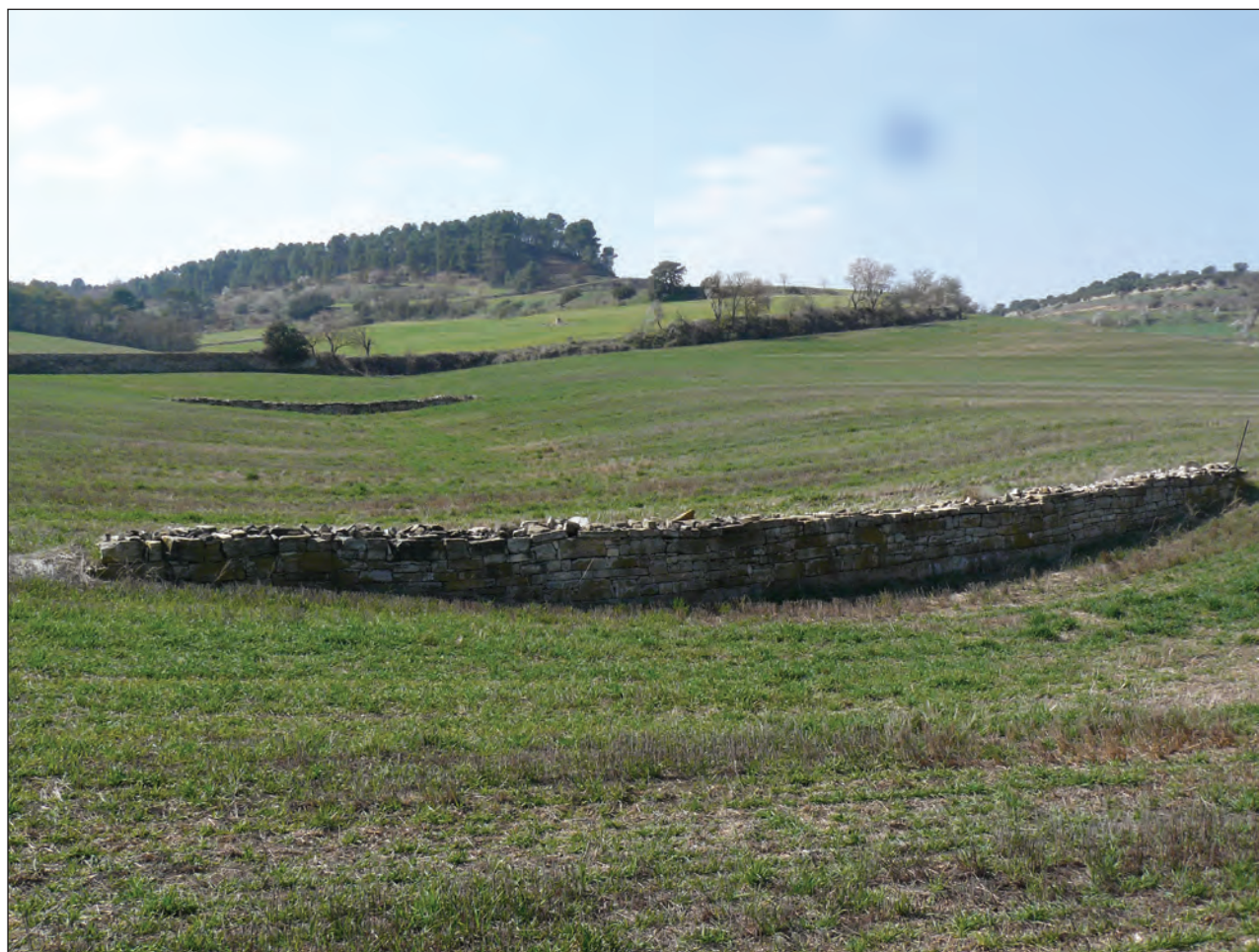
Figure 6: Stone walls built in the 1980s-1990s across a gully.
