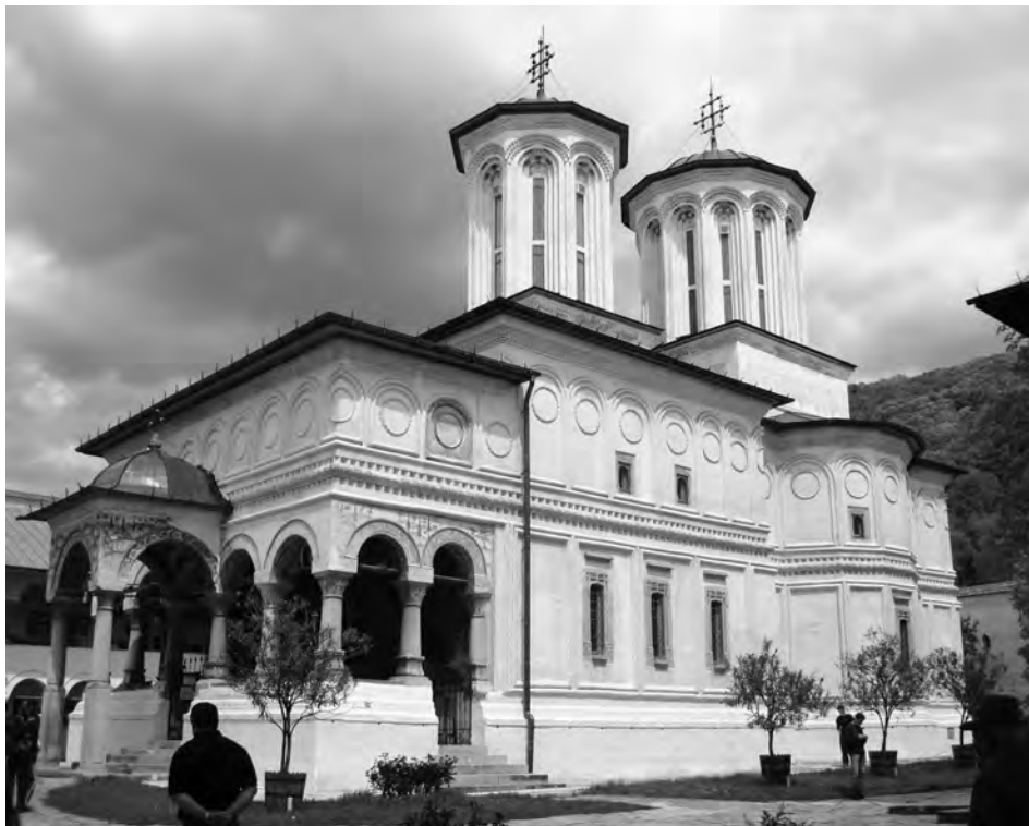
Figure 1: Monastery of Arges in Romania.
