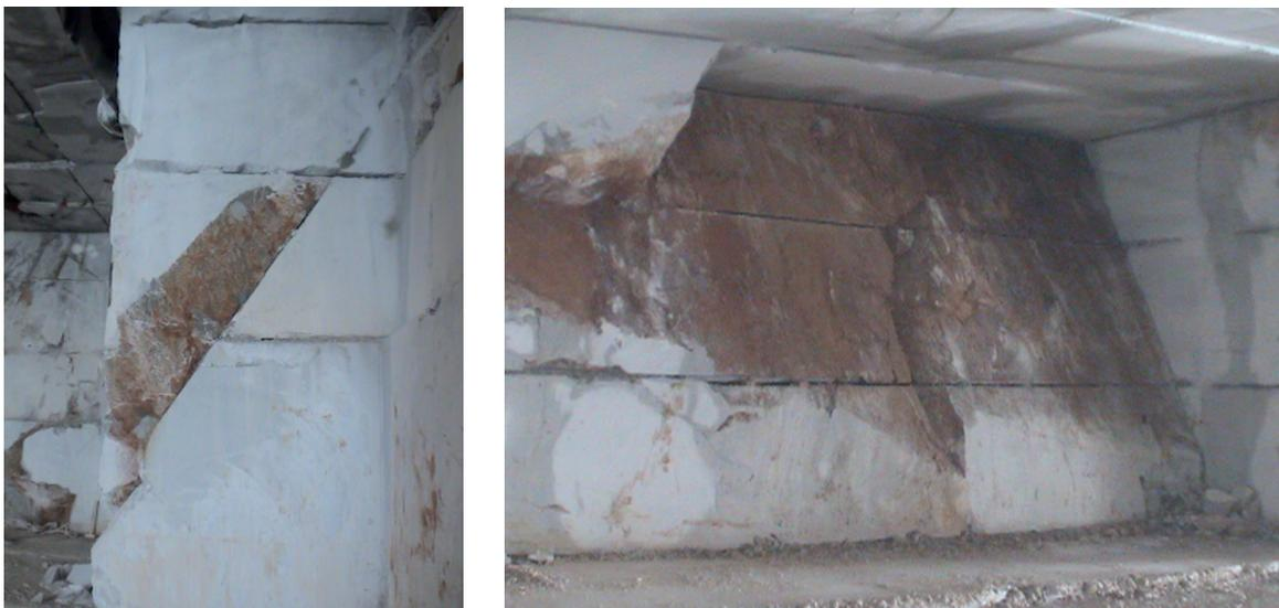
**Figure 2:** Open fissures in underground structures of quarry Lipica II.
