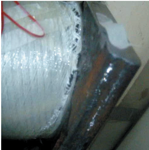
Fig. 14. Failure of the structure in the clamped end under a transverse end load
