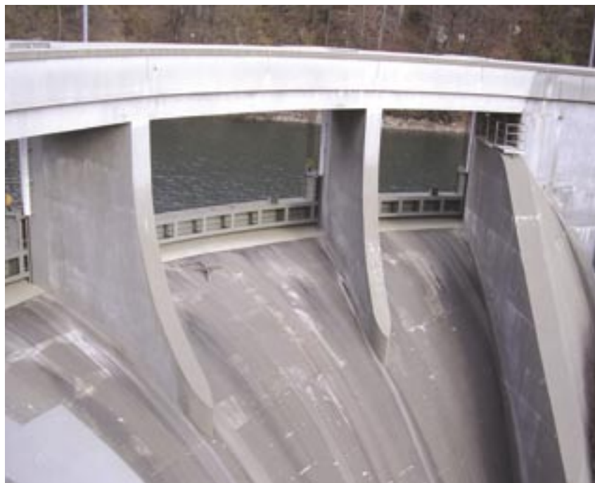
60 m visoka betonska pregrada HE Moste (foto: Aleksandra Privšek).
