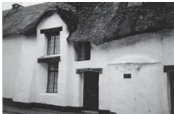
Slika 8: Najbolj znana angleška zgradba iz ilovice, pomešana s slamo v Devonu iz leta 1539. The best known English building made from clay mixed with straw, built in Devon in 1539.
