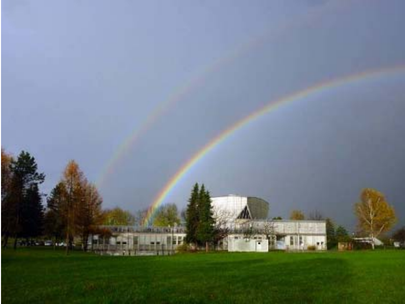
Figure 25: View of the IJS Reactor Infrastructure Centre
