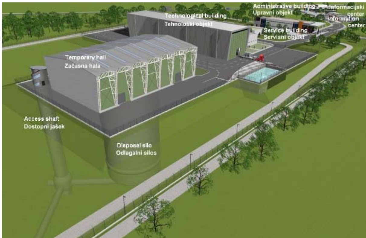
Figure 15: LILW repository facilities as in the Detailed Plan of National Importance for an LILW Repository in Vrbinja in the Municipality of Krško
