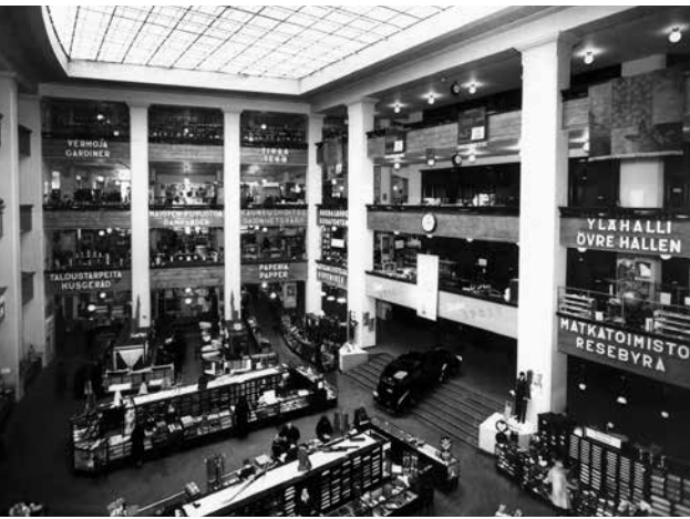
The atrium of the Stockmann department store. Photo: Roos. Museum of Finnish Architecture.
