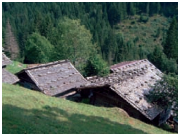
Fig. 18: Traditional wooden shingle roof. Tradiconalna skodlasta streha.
