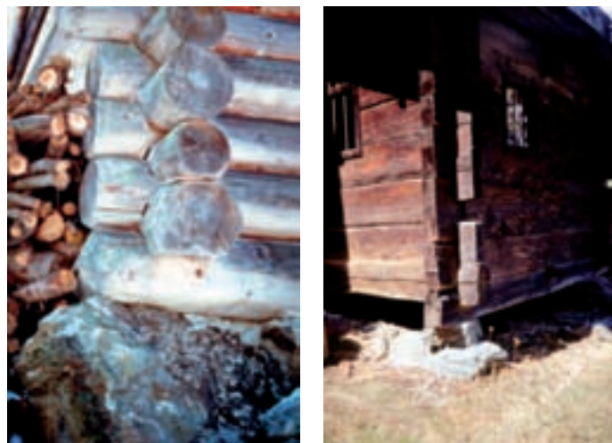
Fig. 5: Example of the use of round (left) and squared (right) logs. Primer uporabe okroglih (levo) in kvadratnih (desno) brun.
