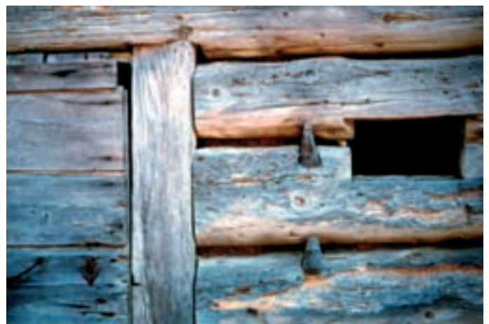
Fig. 24: The window as a small opening between two logs. Okno kot majhna odprtina med dvema bruni.
