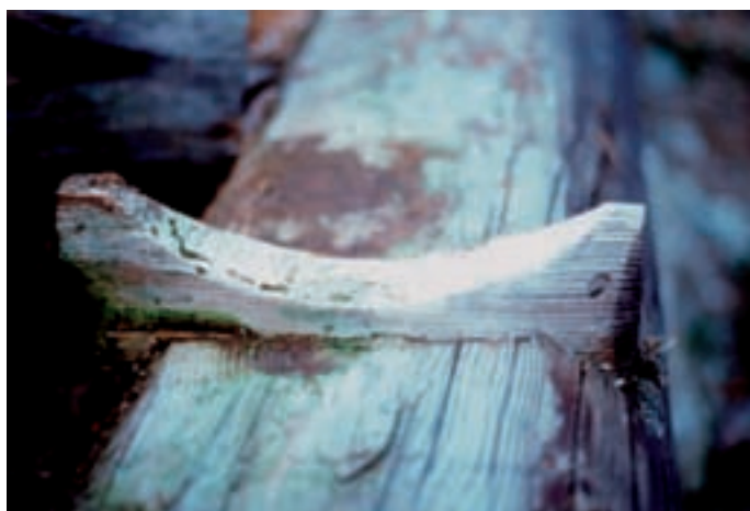
Fig. 10: Detail of the interposition of wooden elements between the logs. Detajl vmesnega lesenega fiksirnega elementa za nalaganje brun.
