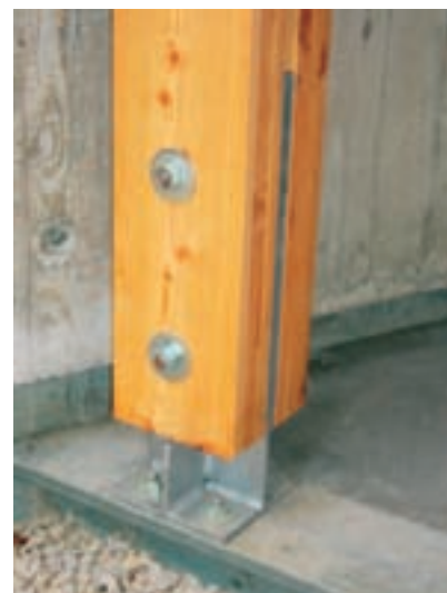
Slika 13: Detajl pritrditve lesenega stebra spodaj (les - jeklo). Detail for fastening a timber column at the bottom (timber - steel).
