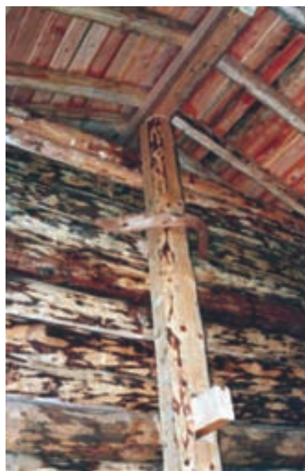
Fig. 17: Detail of pillar locked to the wooden wall. Detajl pričvrstitve stebra na leseno steno.
