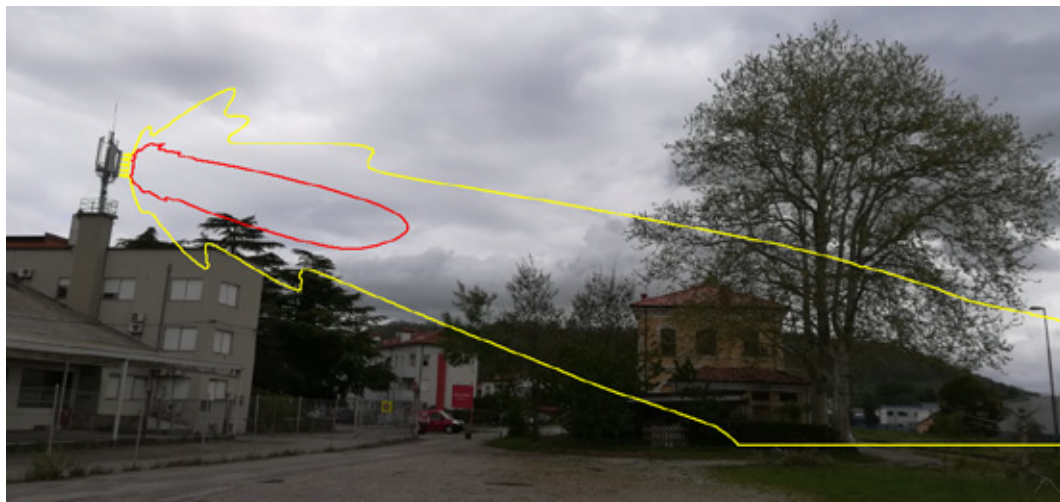
Figure 3.7: Compliance zone for a typical 3G – 5G base station with a 10°downtilt according to Slovenian legislation: yellow for I. area of protection, red, for II. area of protection. Limit values for II. area of protection is similar to ICNIRP guidelines and 1999/519/EC recommendation, for the I. area of protection, the limit values are 10 times lower (for power density).
