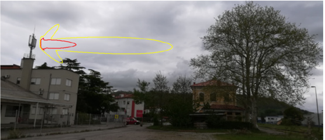
Figure 3.5: Compliance zone for a typical 3G – 4G base station according to Slovenian legislation: yellow for I. area of protection, red, for II. area of protection. Limit values for II. area of protection is similar to ICNIRP guidelines and 1999/519/EC recommendation, for the I. area of protection, the limit values are 10 times lower (for power density).
