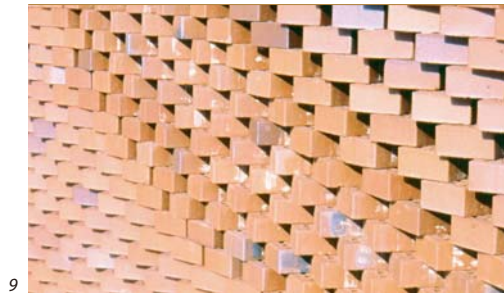
9 Slika 9: Opečnati zid, ki ga je naredil robot, Studio Fabio Gramazio, Matthias Kohler, ETH Zürich Figure 9: Robot-laid brick wall, Studio Fabio Gramazio, Matthias Kohler, ETH Zurich.
