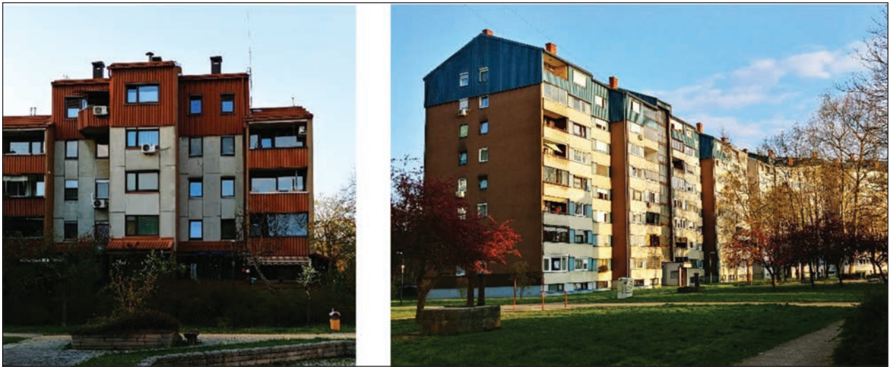
Figure 2: Modular construction of the residential neighbourhood Fužine from the 1980s in Slovenia, consisting of prefabricated sections of the façade, prefabricated wall panels and interior partitions (Photo: Simon Petrovčič, 2020).
