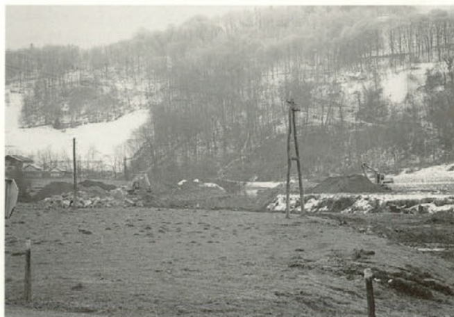
Regulacija Dravinje pod mostom v Slapah – december 1996
