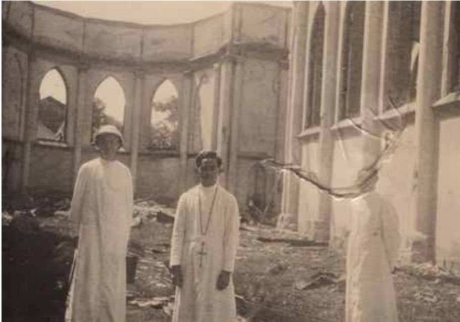
Figure 2: The ruin of the same Church building in 1945 (Source: Archives of the Provincialate of the Congregation of the Mission, Surabaya, Indonesia).
