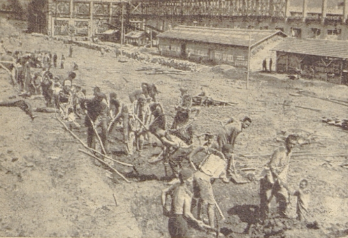
Youth builds copper rolling-mill at Sevojno (Serbia)
