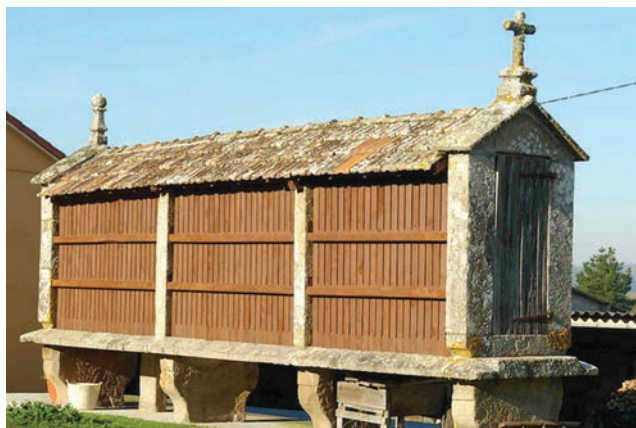
Slika 6: Hórreo iz lesa in kamna na več zidcih. Amoeiro, Spain. [www.horreosdeg Galicia.com] Figure 6: Mixed hórreo on dwarf walls. Amoeiro, Spain. [www.horreosdeg Galicia.com]
