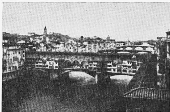
Bridges Vecchio — Trinita — Carraia
