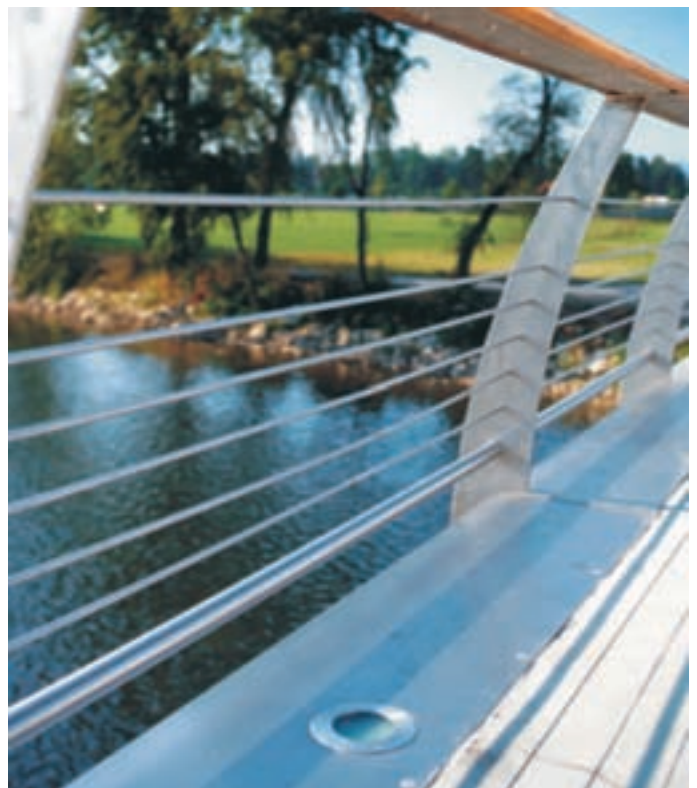
Slika 7: Mostna ograja ima široko mostno polico in niz svetilk, skritih v zaključnem vencu objekta. (foto Miran Kambič) The bridge parapet has a wide bridge shelf and rows of lights hidden in the bridge's concluding cornice.
