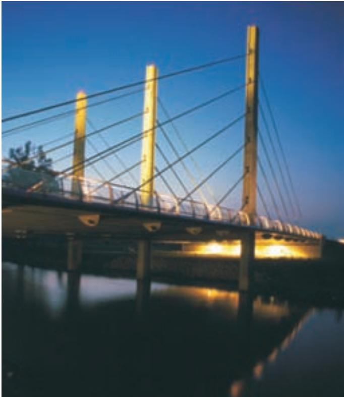
Slika 4: Prehodnost podmostja omogoča tanka, le 40 cm debela mostna plošča. (foto Miran Kambič) Permeability of the bridge's undercarriage is enabled by a slight, only 40 cm thick bridge plate.
