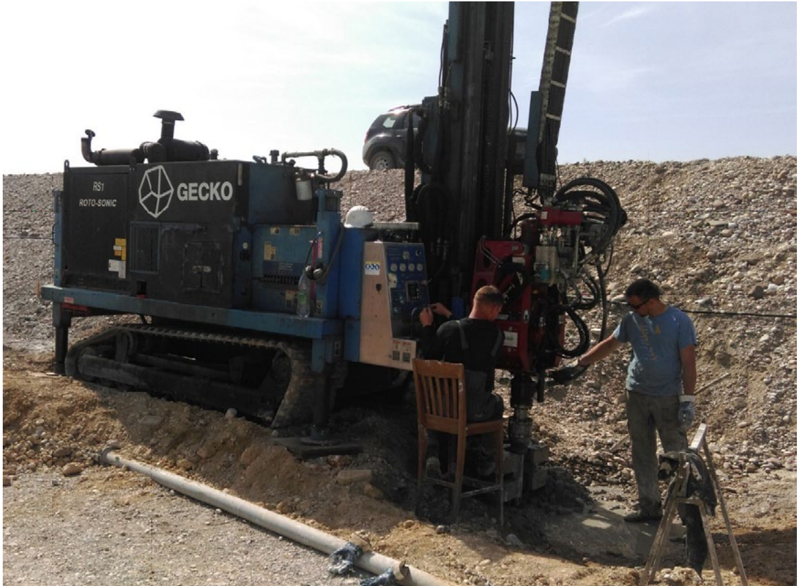
Figure 5. Drilling equipment fitted with a high-frequency drill head (source: Gecko Ltd.).
