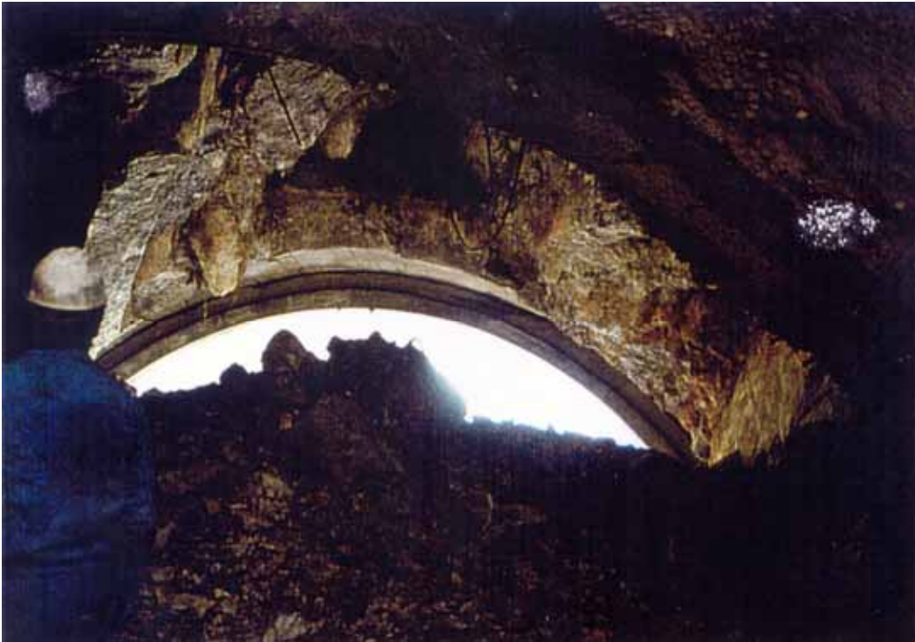
Figure 5. Slide of a dolomite block in the Golo rebro Tunnel at chainage 27+974 [2] Slika 5. Zdrs dolomitnega bloka v predoru Golo rebro na stacionaži 27+974 [2]
