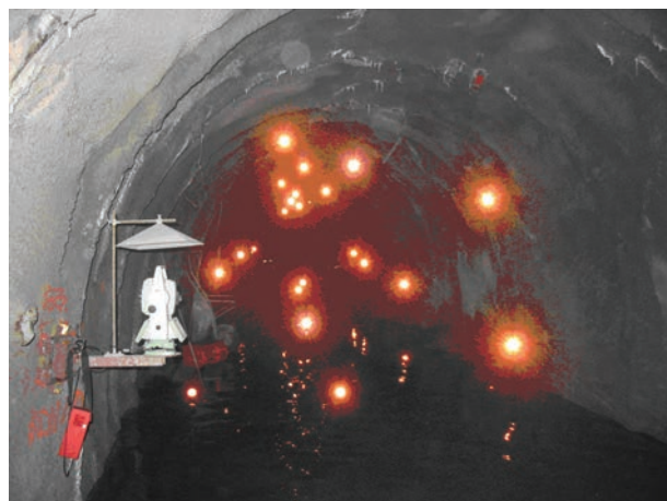
Figure 11a. Electronic tachymeter and geodetic prisms installed in the primary lining and on the bottom of the exploration gallery.
