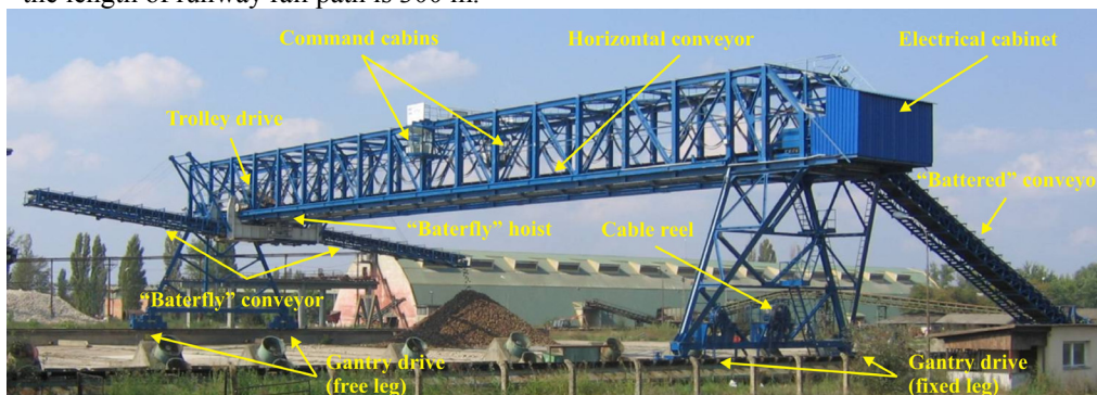
Fig. 6. Gantry crane with indicated drives
