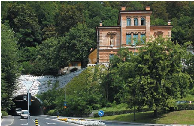
A secession villa above the tunnel under the Ljubljana Castle, Karlovška 3, where interviewers were crowded during the 1961 population census and where later on the Register of Territorial Units and the Register of Organisations and Communities were operating.
