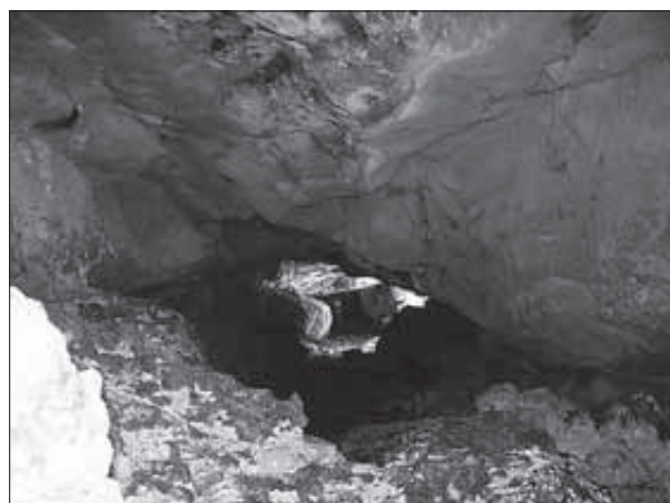
Fig. 13: Zulum overflow gallery. (Photo: A. Iurkiewicz).
