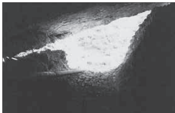
Fig. 20: Betas entrance and water pipes. (Photo: Z Stevanović).
