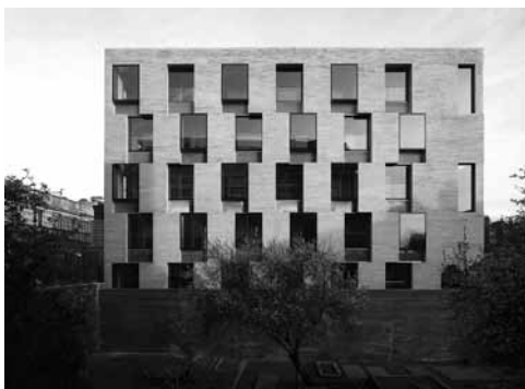
Zahodna fasada, 450 mm debel zaslon, ki daje občutek debeline kamna. The west elevation, the 450mm deep screen, which makes you feel the depth of the stone.
