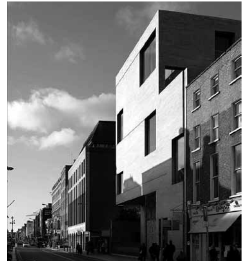
Zgradba oddelka za finance posreduje med sistemom ulice in sistemom trga. Finance Department building mediates between the street system and the square system.
