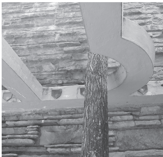
Slika 7: Fallingwater – spoštovanje narave, betonska pergola se je umaknila drevesu. Figure 7: Fallingwater – respect for nature: concrete pergola was withdrawn to avoid the tree.
