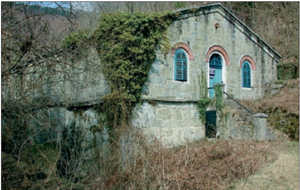
Fig. 4.: At Gornje Ležeče there are two water reservoirs, which could contain more than 20,000 m 3 of water. Picture presents the south water reservoir at Gornje Ležeče that could contain 14,000 m 3 of water (Photo: N. Ravbar).
