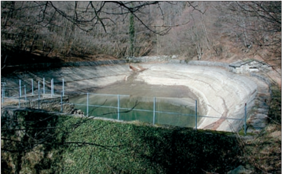
Fig. 3.: For the needs of the steam railway several superficial streams were captured at the contact of karst with flysch (Photo: N. Ravbar).
