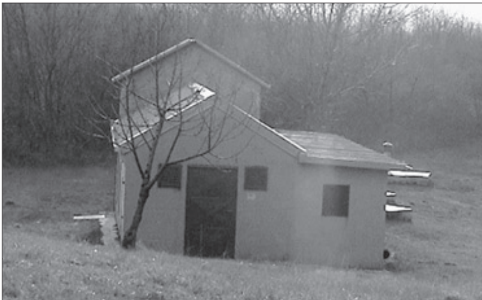
Fig. 6.: Drinking water supply of today is mainly based on karst groundwater pumping near Klariči (Photo: N. Ravbar).
