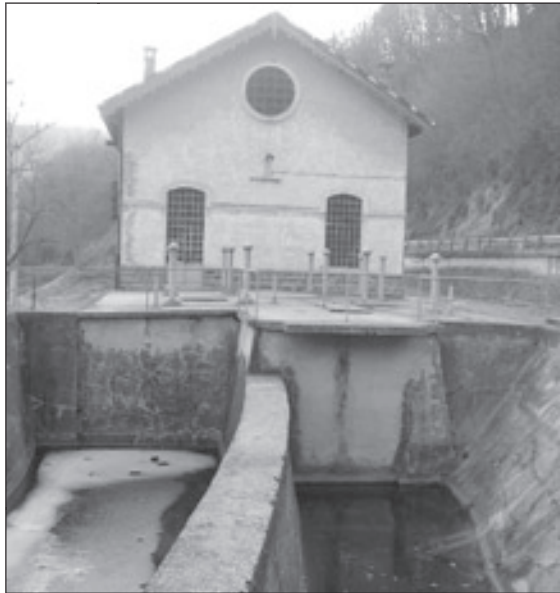
Fig. 5.: When the needs for water increased rapidly, an additional water pumping station was built (Photo: N. Ravbar).
