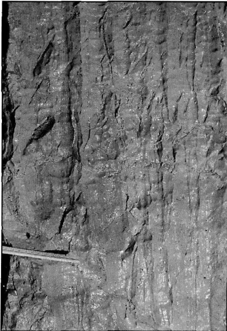
Fig. 8: The shafts wall shaped by trickling water
