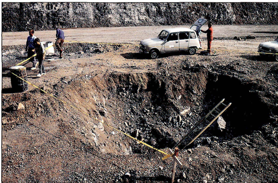
Fig. 8: Collapse above a cave Sl. 8: Udor nad jamo
