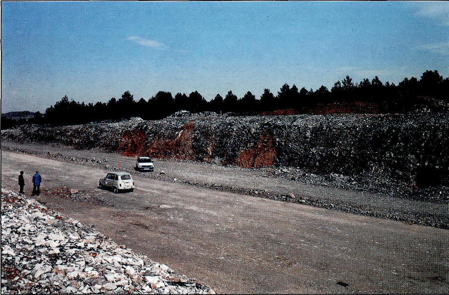
Fig. 5: Caves, filled with sediments on a slope of a cutting Sl. 5: Jame, zapolnjene z naplavino, na brežini useka
